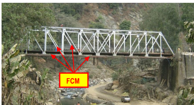
Fig.1: Typical Example of Fracture Critical Member
